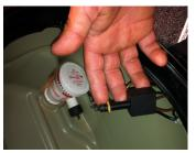
Trim the black switch wires as close as possible to the old switch. Cut the old wire connector out of the line by cutting the two black wires that lead in to it as close to the wire connector as possible.
