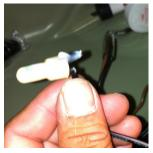
Next you will install the new switch. Cut the black wires leading out of the new switch to approximately 6 and 10 inches respectively. Strip away the black cover at the ends of these wires leaving about ¼ of an inch of silver wire exposed. This will leave you with 4 exposed black wires.
